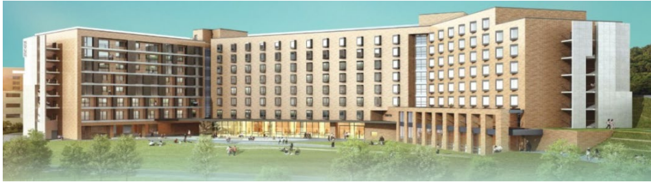
Figure 2. Chejung House (near East Gate)
